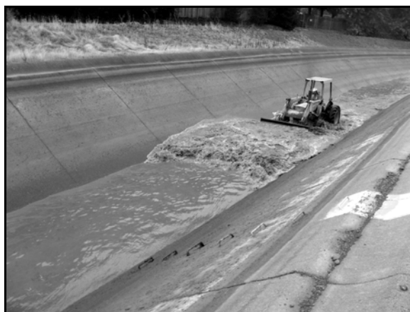
Figure 3. Pushing sediment and vegetative detritus down Union Check at MP 14.80. Photo of November 3, 2006.
