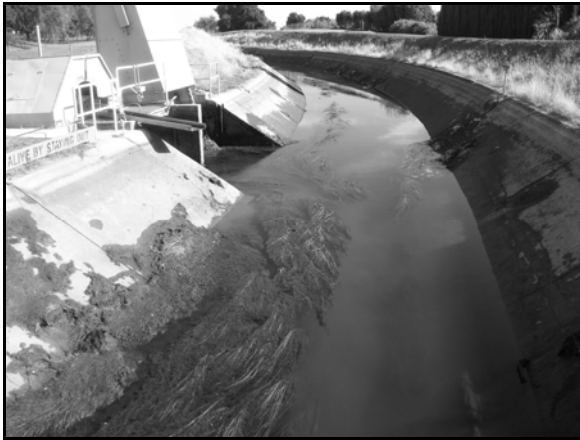
Figure 4. Thick growth of algae and macrophytes that plug the intake to the Waterman WTP located just upstream of Serpas Check. Photo of November 9, 2006.
