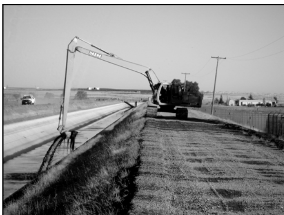
Figure 2. Removal of aquatic weeds and sediment from Sweeney Check at MP 6.15. Photo of October 19, 2006.
